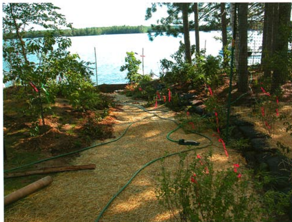
Figure 2. Hvam site on Found Lake after shot; straw matting with native seed mix woven in replaces boat access and other erosion control and native species plantings in 2008 field season.
