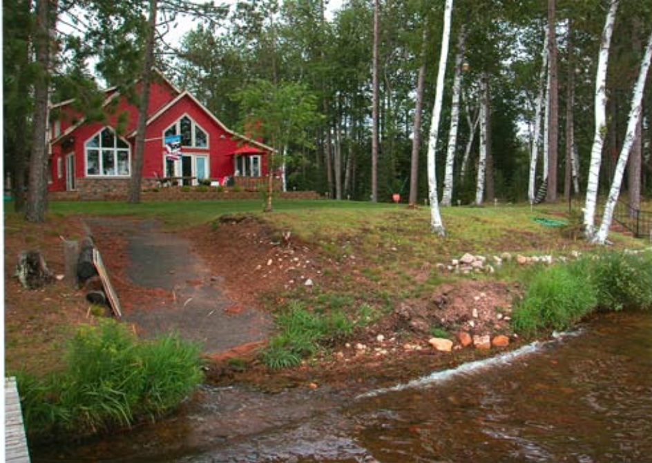
Figure 1. Hvam site on Found Lake before shot; notice spotty turf grass, exposed soil, and erosion problem caused by asphalt boat access.
